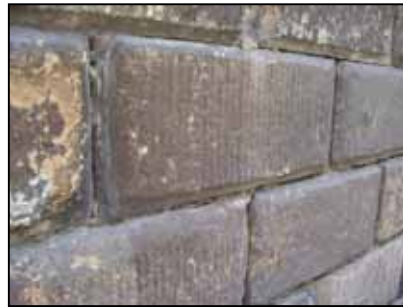
Figure 8. Croste nere in un muro grezzo esterno - Black crust in an external unpolished wall.
